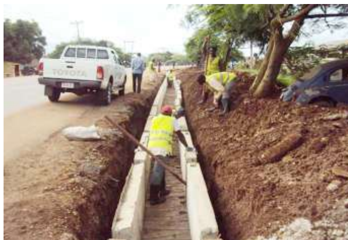
Construction of Precast reinforced concrete drains between CH53 + 359 - CH. 53 + 365 RHS - Ogoja -Ikom Road
