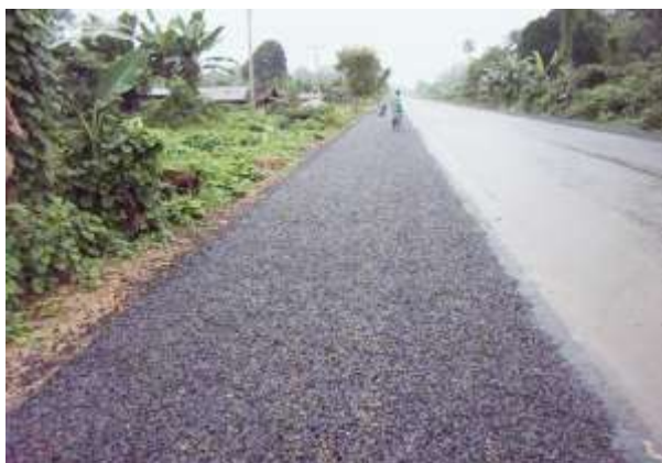
Surface dressing of carriageway shoulders between CH. 55 + 825 - CH. 57 + 300 (RHS) - Abakaliki - Imbok Road
