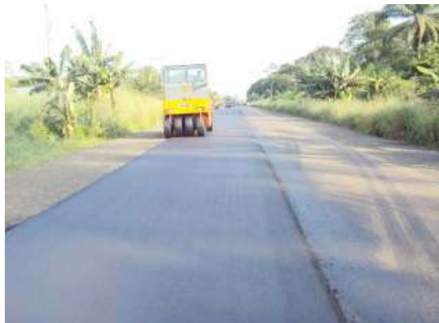
Laying of Asphaltic Concrete Wearing Course around CH. 61 + 870 - 62 + 938 LHS - Abakaliki - Imbok Road
