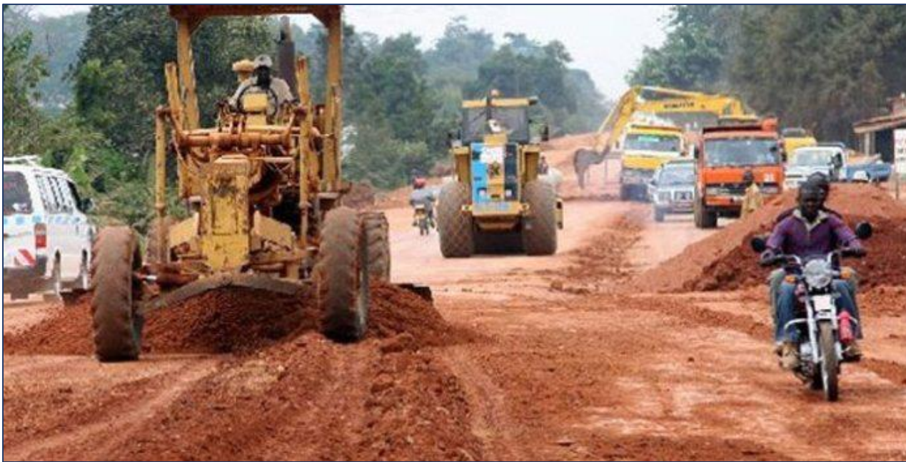
Construction of new roads
