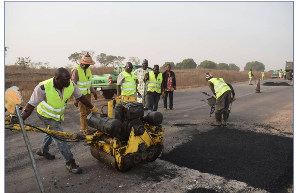
Road Repair Works by FERMA
