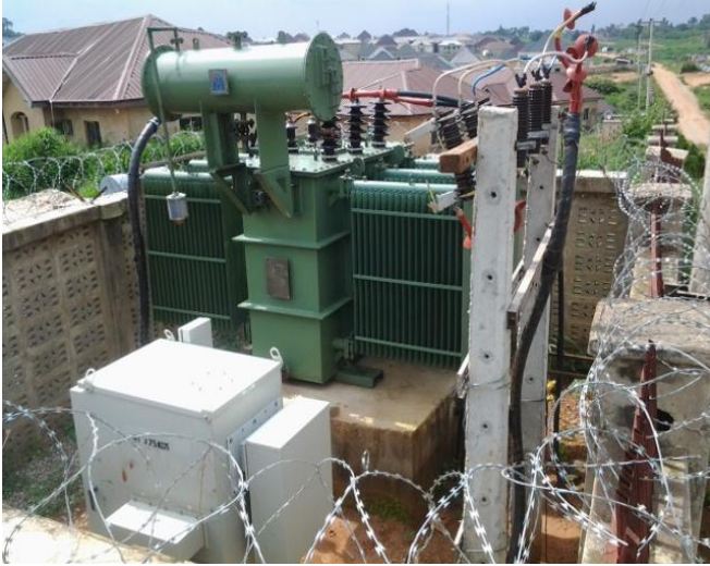
New installed 2.5 MVA substation
